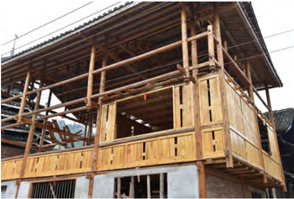
The internal structure of Kam houses
